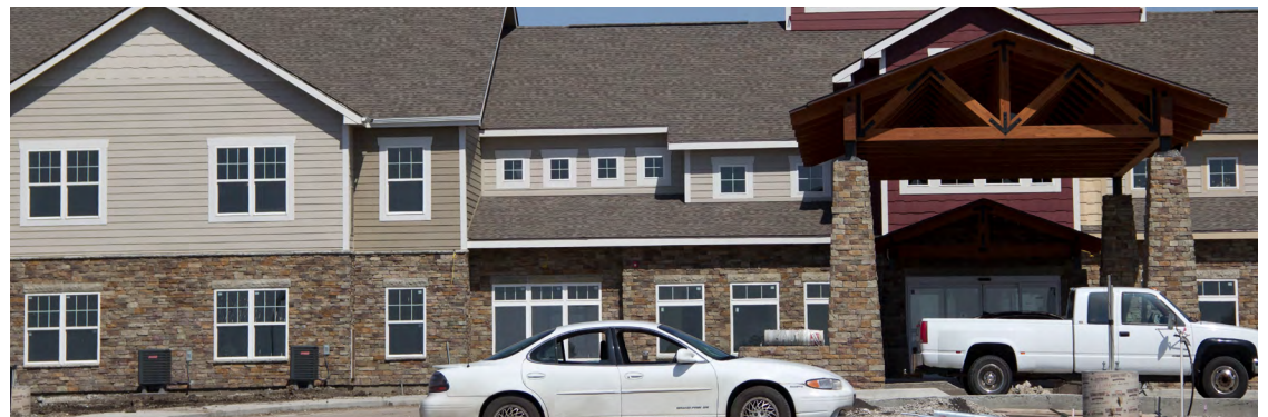
SENIOR CAMPUS - PROVIDES INDEPENDENT, SUPPORTED, AND ASSISTED LIVING OPTIONS IN ONE PLACE WITH COMMON AMENITIES AND MEETING SPACES.
