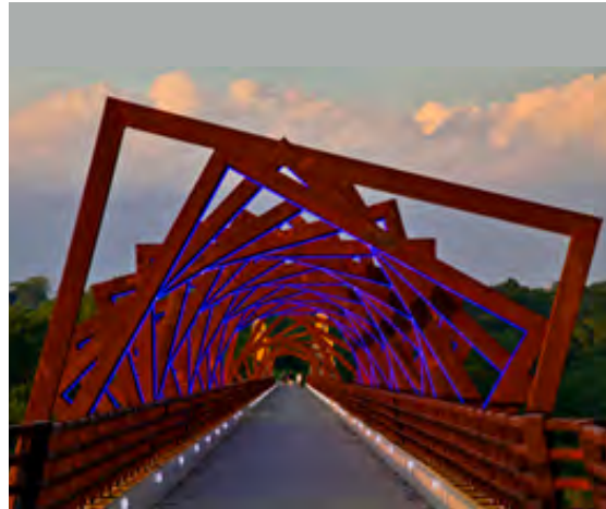
HIGH TRESTLE, CENTRAL IOWA
